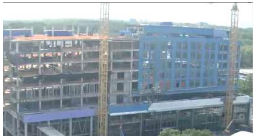
View of construction as of August 2016
