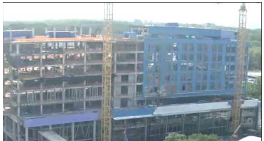
View of construction as of August 2016
