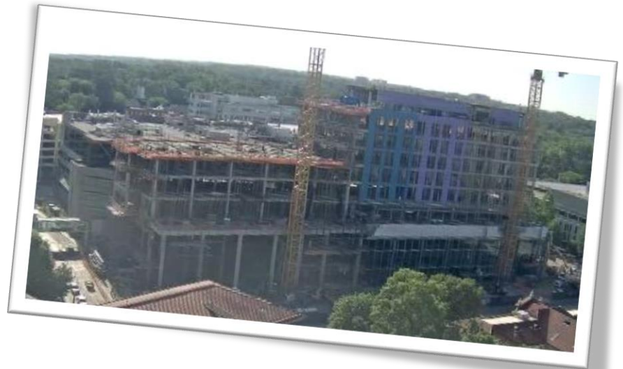
Aerial view of construction as of May 2016.
